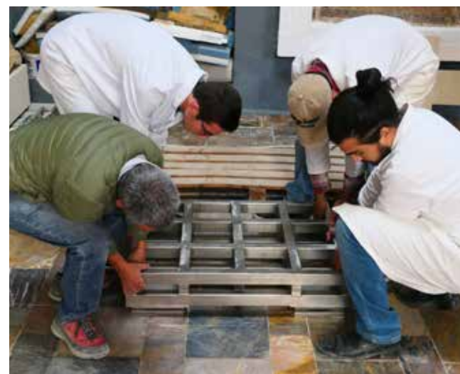
Left: Installing the pedestal for the statue of Apollo with its special earthquake-proof elements. Right: The statue of Apollo on its new pedestal: the inner metal framework is encased by limestone (Photos: U. Kreiling)
