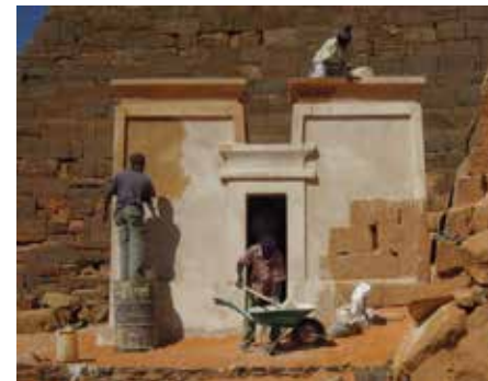
Conservation work at Meroe has many facets, among them delicate conservation and restoration of colored sand stone relief scenes ( right ) (Photo: D. Rütt) and maintenance of reconstructed chapel walls and roofs ( left ) (Photo: T. Bunk)
